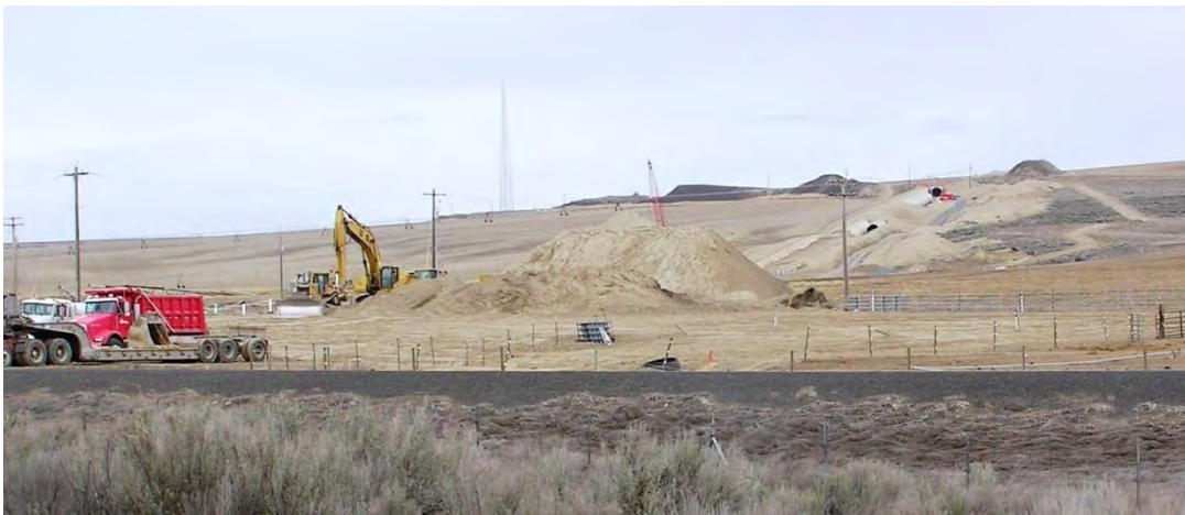
Figure 17c USBoR—Weber Siphon at I-90
