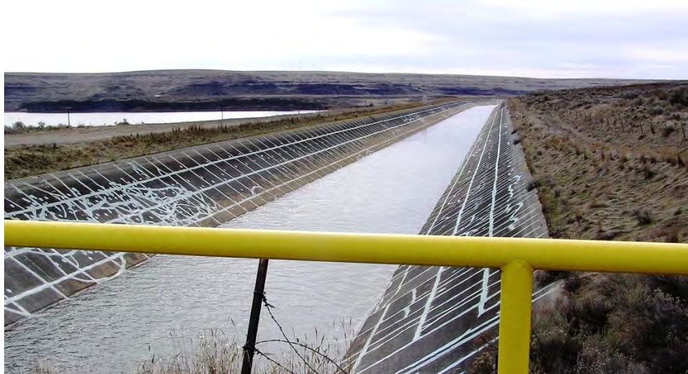
Figure 16 USBoR Main Canal—Pinto Dam at Billy Lake
