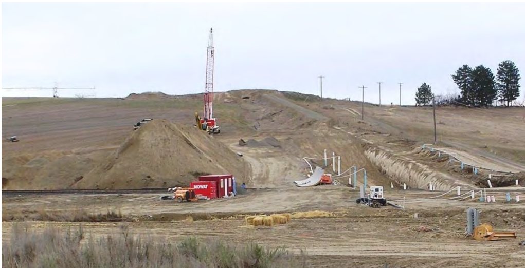
Figure 17d USBoR—Weber Siphon at I-90
