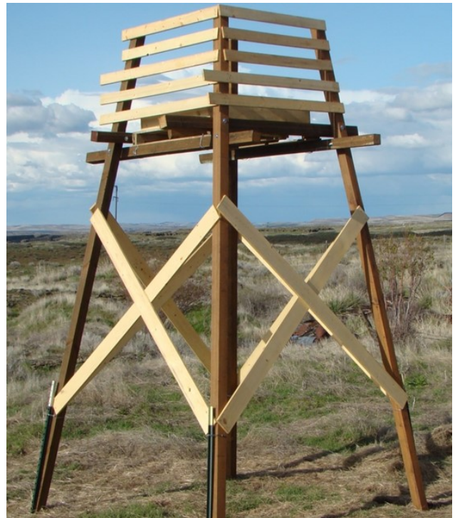
The nesting platform was completed on April 9, 2015 with the installation of wind break panels.
